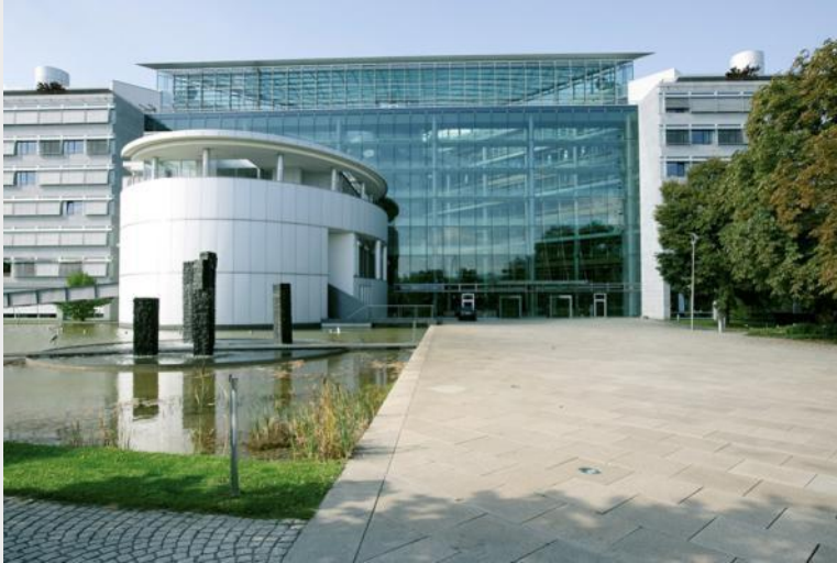
Boehringer Ingelheim Center Our headquarters in Ingelheim, Germany
